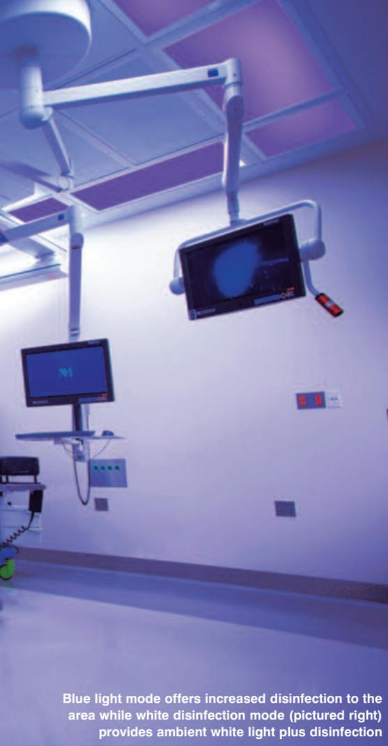
Blue light mode offers increased disinfection to the area while white disinfection mode (pictured right) provides ambient white light plus disinfection
